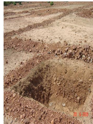
Fig 6: Pit made on upland with less than 8% slope
